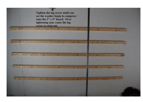
Once you are completed you should have six (6) 2" x 4" x 12" boards lag screwed to the ceiling joists on 16" centers from each other. Now you can begin to layout where you want to mount the garage lift drive frame.
