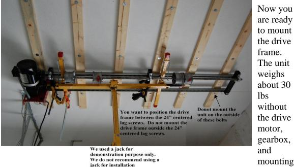
the drive frame. The unit weighs about 30 without the drive motor, gearbox, and mounting plate.
