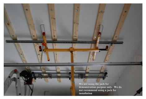
If you are remote mounting the drive then you will need to install two cable support brackets. Follow the same procedure spelled out for mounting the drive unit but measure from the side of the cable drum closest to the electrical box to the first cable support bracket. Then measure 48" from this point for the second cable support bracket.
